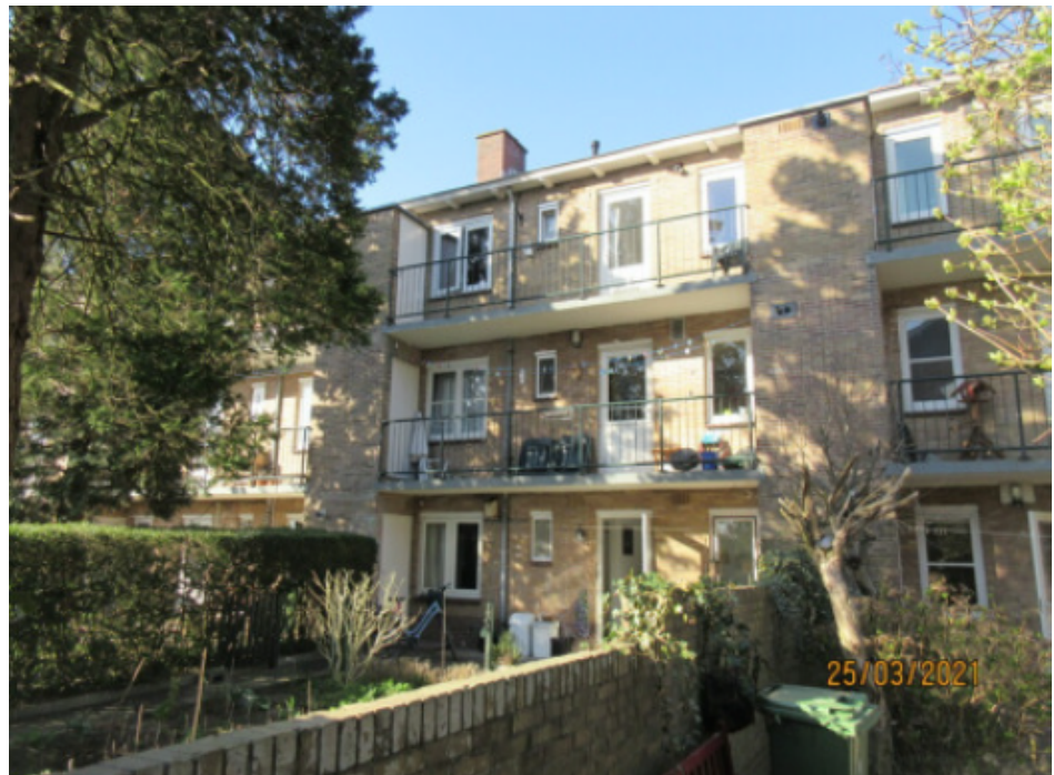
Project in Hilversum
